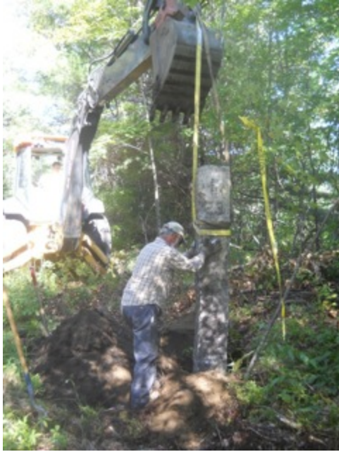
Crew from D. R. Key easing eight-foot 1400 lb. granite mile marker into place along the rail trail near Mirror Lake in Canaan.
